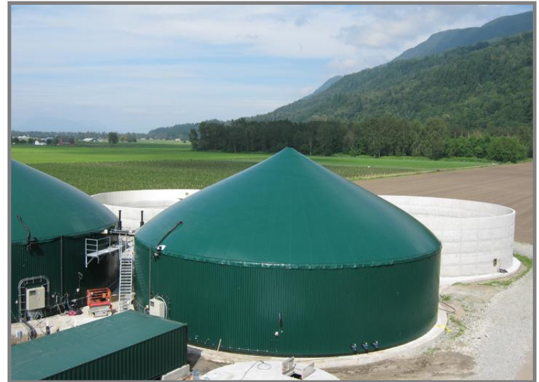
Catalyst Power Anaerobic Digester
