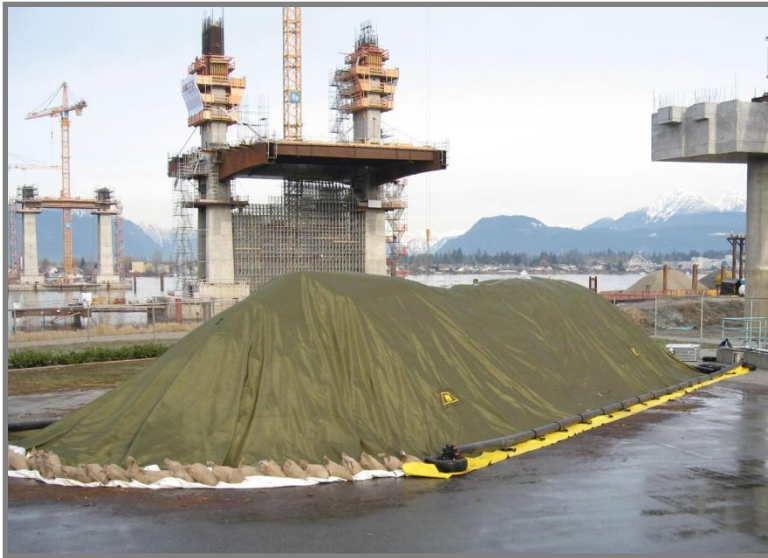
2008 Metro Vancouver Gore Cover Project
